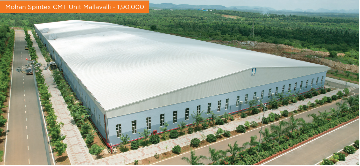
Mohan Spintex Boiler and husk shed Mallavalli
